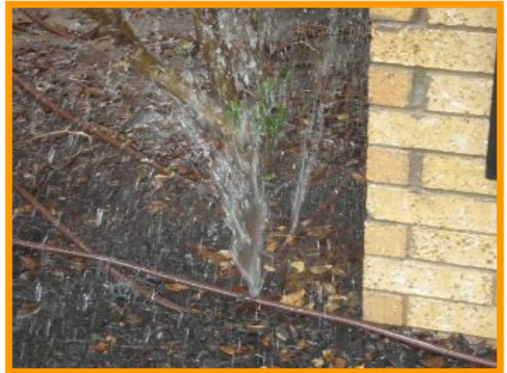
** High Priority Item ** Damaged sprinkler drip lines are allowing geysers of water to shoot up at front flower bed on station/ zone 5. Repairs are needed.
